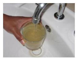
This is due to old iron plumbing inside your home. You can run your faucet as needed to bring in fresh water from the water main, purchase a water filter, or consider replacing your pipes. Contact the Water Quality Line and ask for a water test kit that includes testing for iron. Iron is an essential nutrient and is not a health risk.
