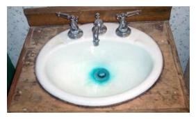
This is commonly caused by new copper plumbing or existing copper plumbing that is corroding. Run your faucet as needed to bring in fresh, uncolored water from the water main. Contact the Water Quality Line and ask for a water test kit that includes testing for copper. Copper is an essential nutrient, but it can be harmful in large doses.
