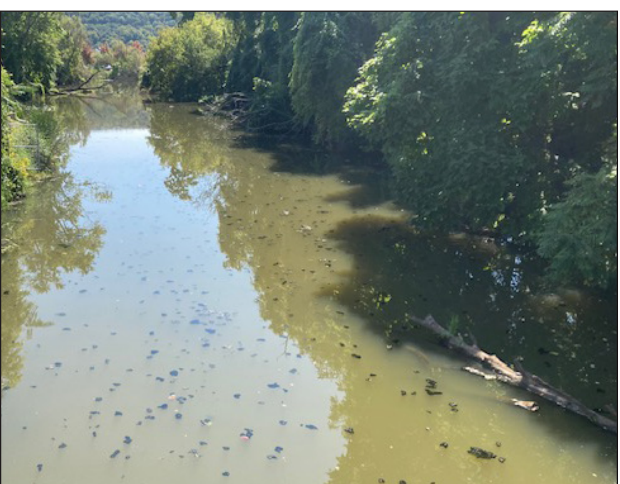
Flood Control Channel between Wegmans and Nate's Floral Estates in the City of Ithaca on 9/5/24
