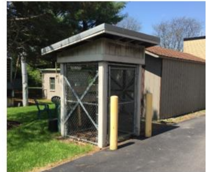
Fenced structure with cooler: The door to the structure will be unlocked. Please close the door after depositing the sample.
