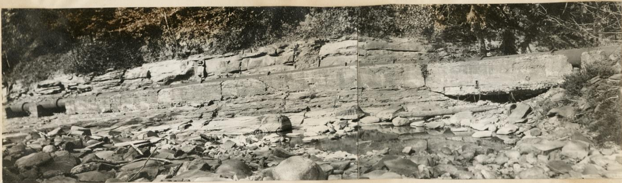
View of 30' Dam 24" Pipe line around turn above Van Natt's, showing foundation washed out by flood.
