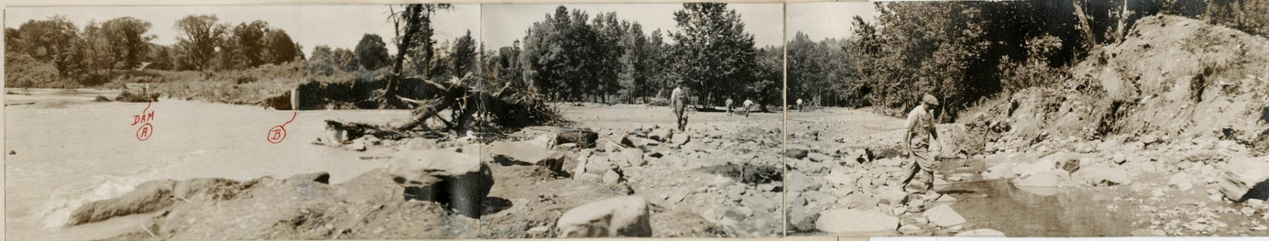
View looking northwest, showing top of Silt Dam "A" and "B", and embankment, left, which was protected by the core wall.
